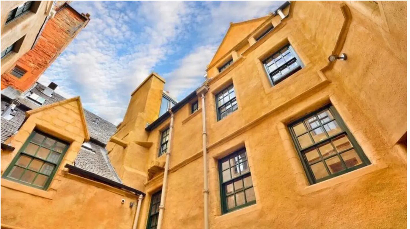
Restored Patrick Geddes Centre for Learning and Conservation
