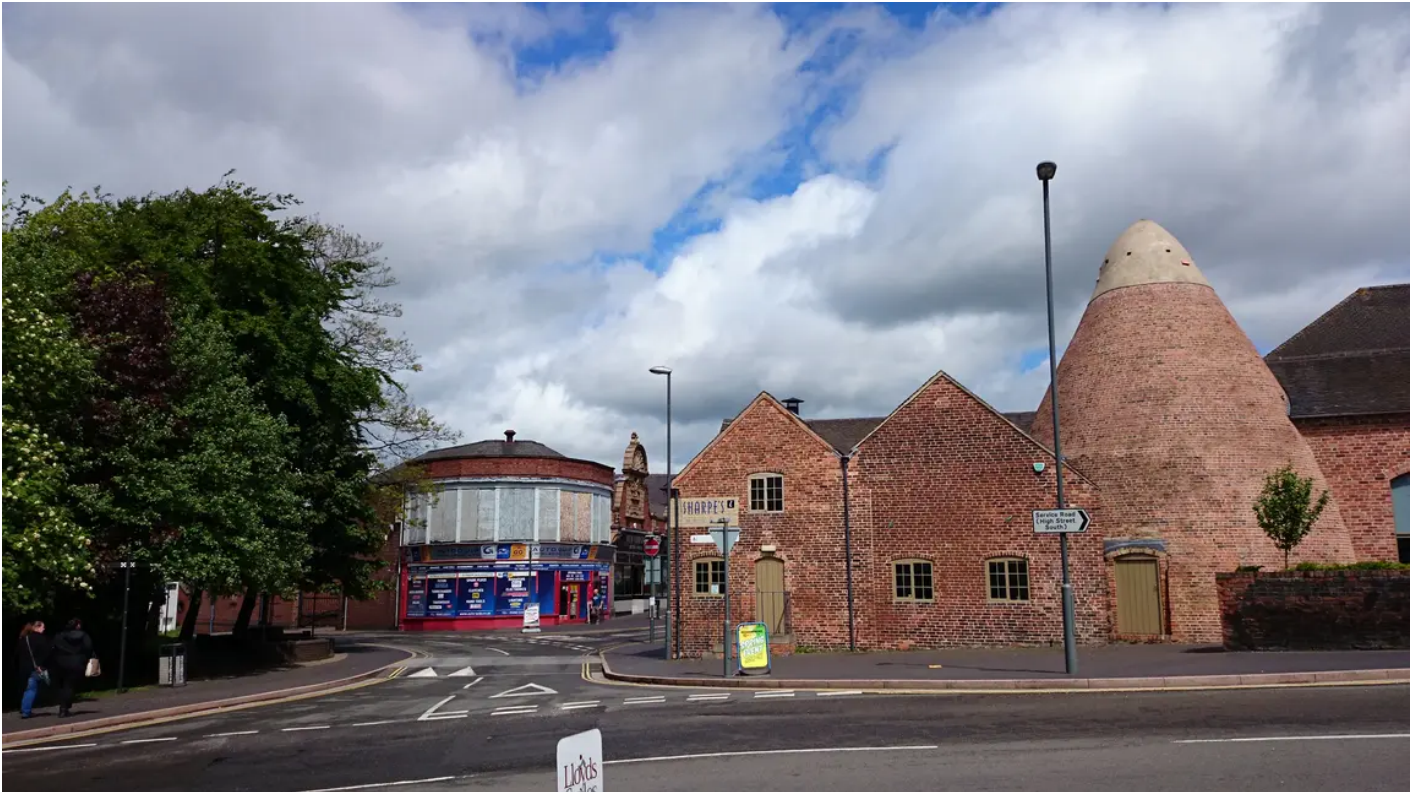
West Street, Swadlincote Town Centre
