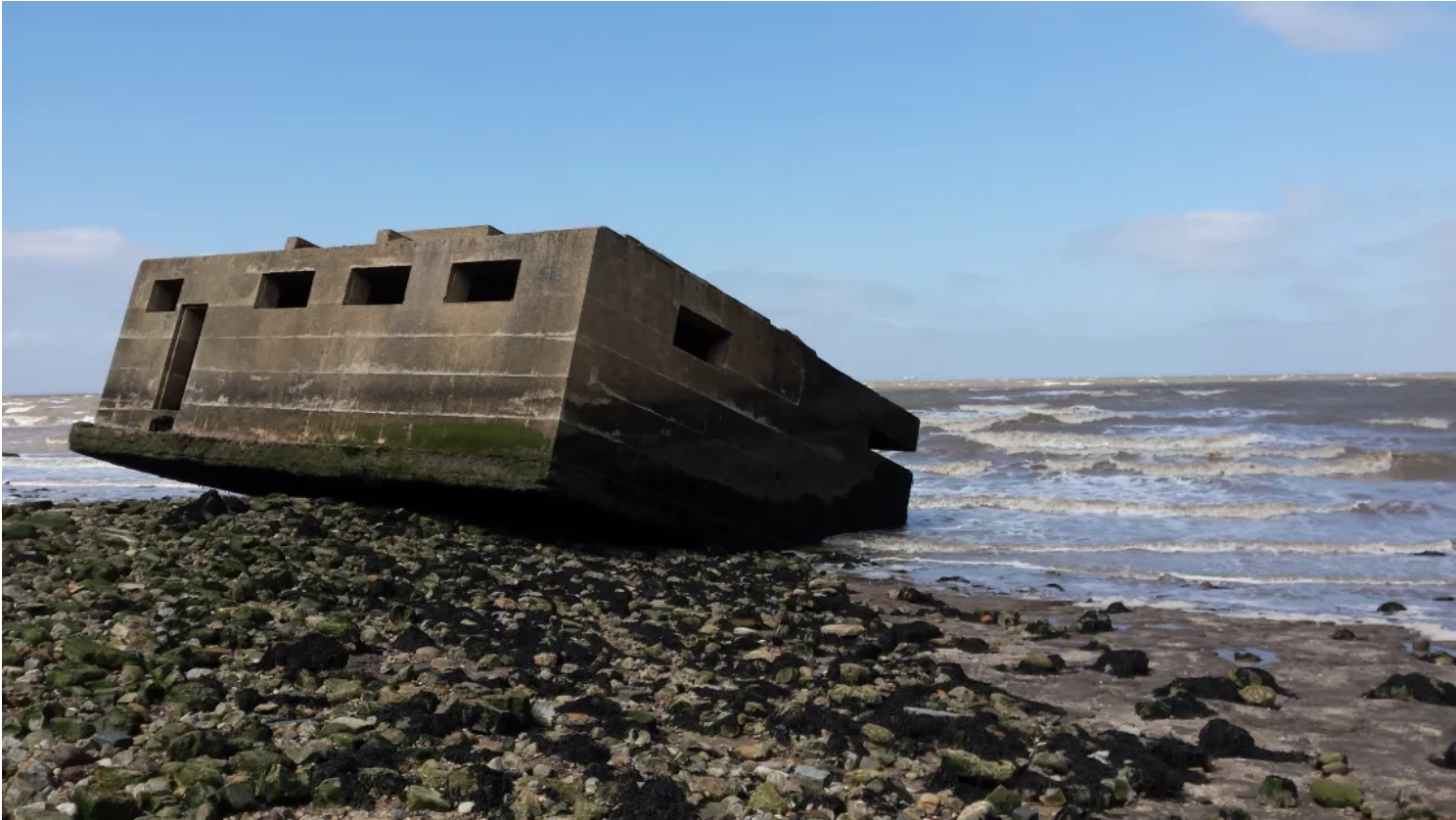
Pill box disappearing in to the sea on the Isle of Sheppey CITiZAN
