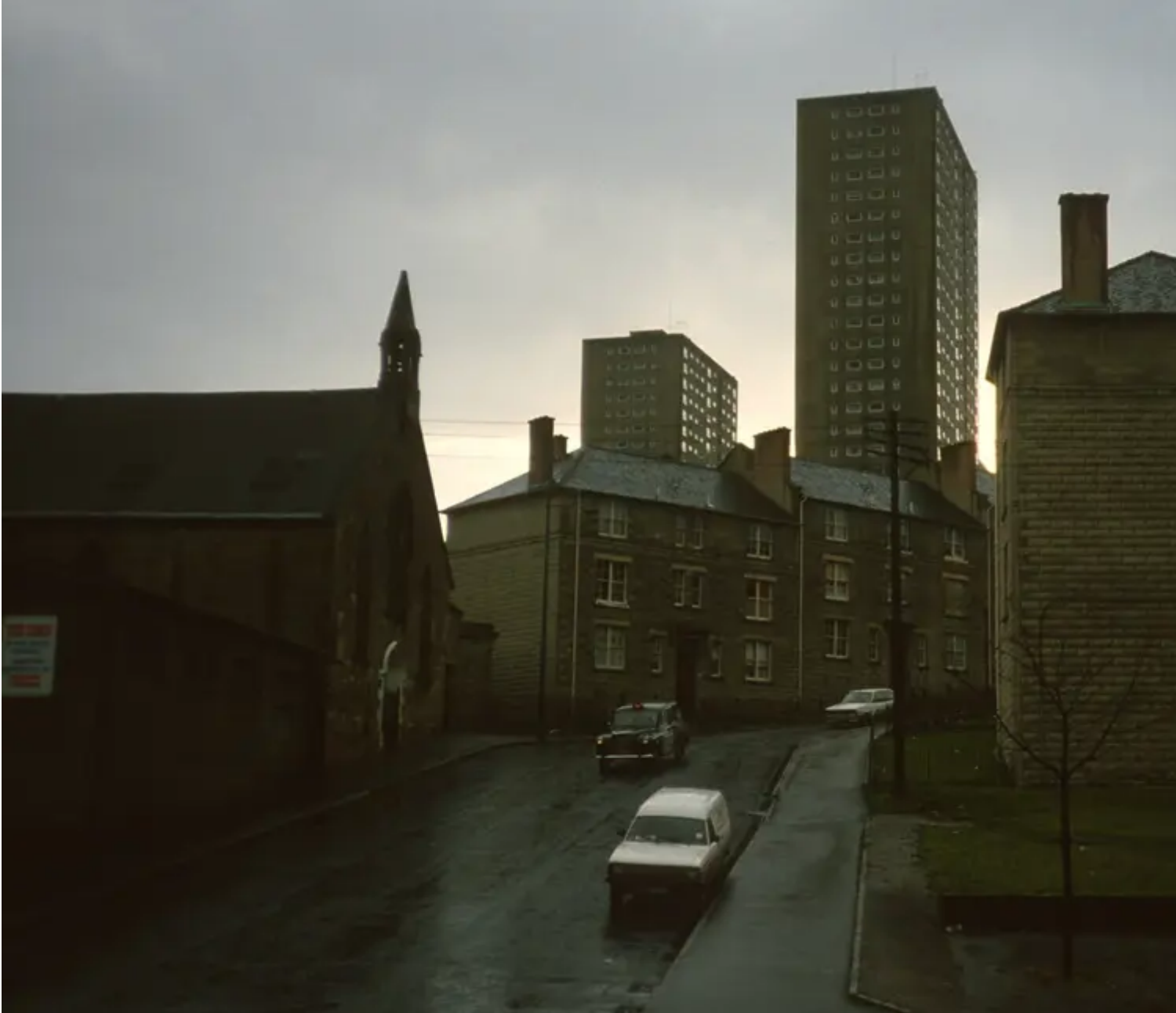
Royston B in Glasgow, shown in its partly-demolished state
