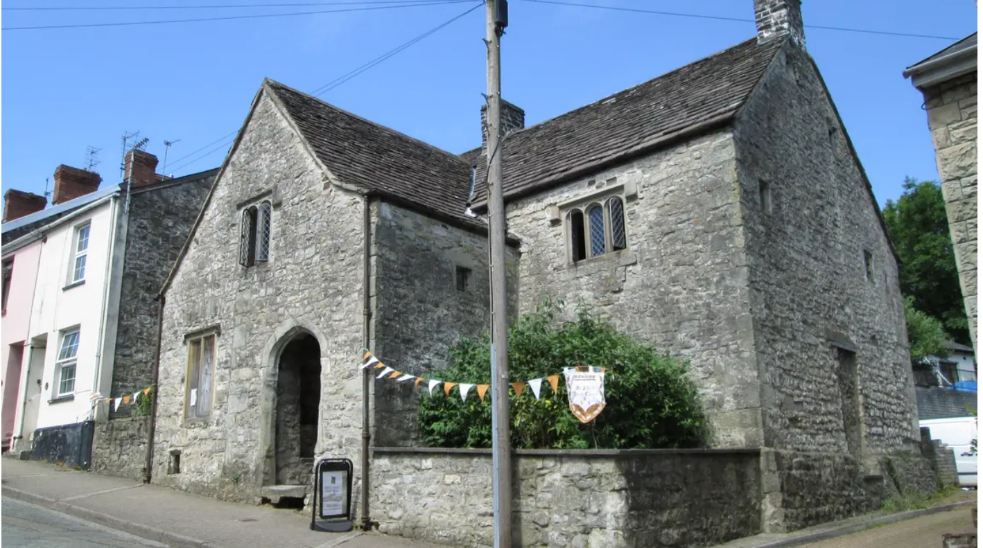
St John's House, Bridgend
