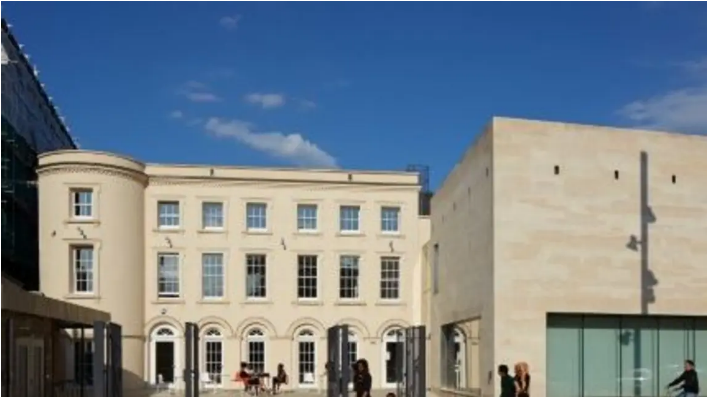
Outside view of Black Cultural Archives building in Brixton
