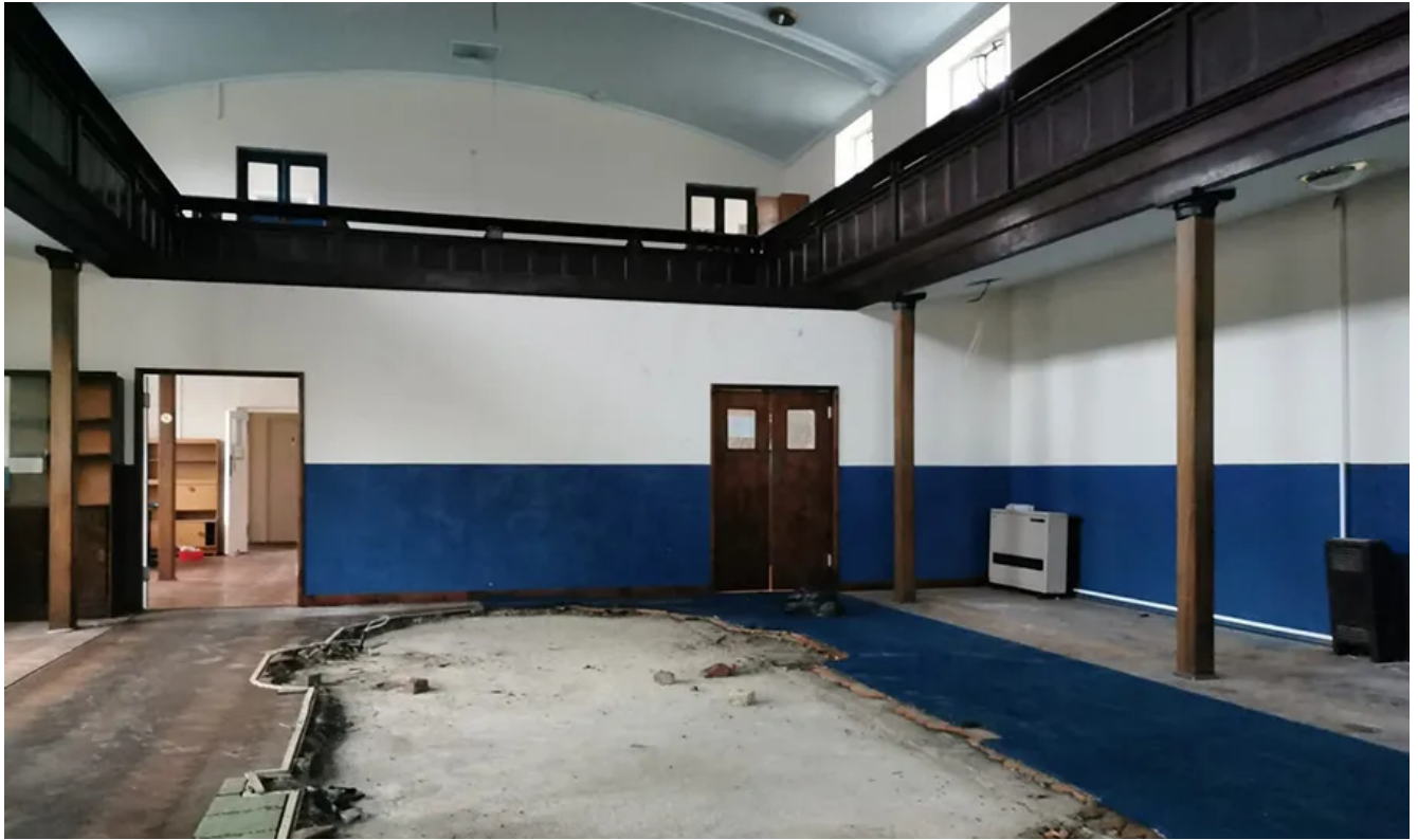
The synagogue was lying empty before ARK took over the building. Credit: Nathan Jones.
