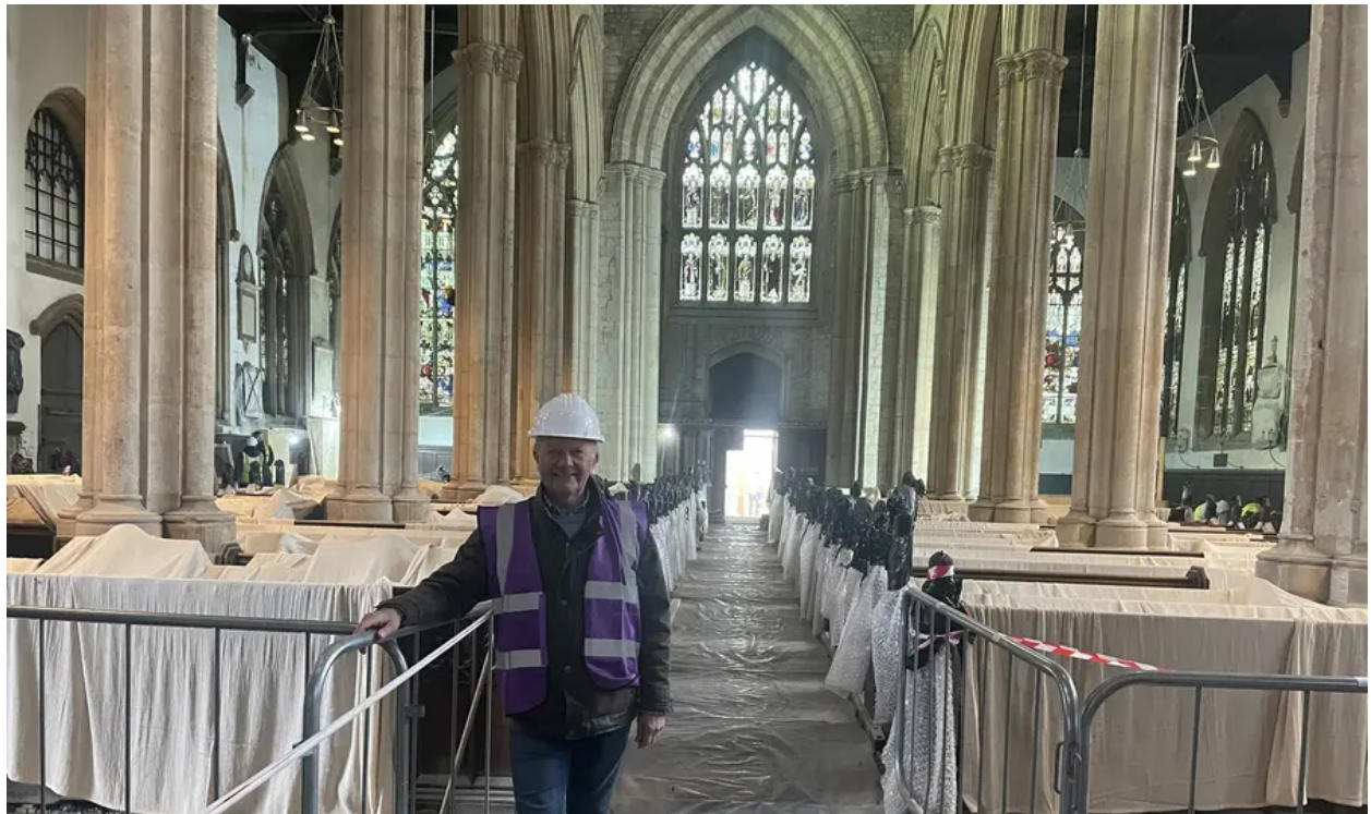
Churchwarden and Project Lead Andrew Fearn examines the work in progress at St. Mary Magdalene, Newark.
