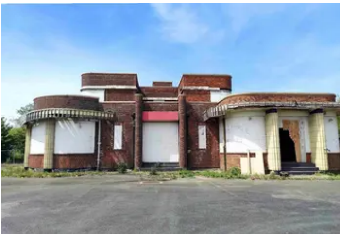
The Iron Duke before restoration . Credit: Great Yarmouth Preservation Trust.
