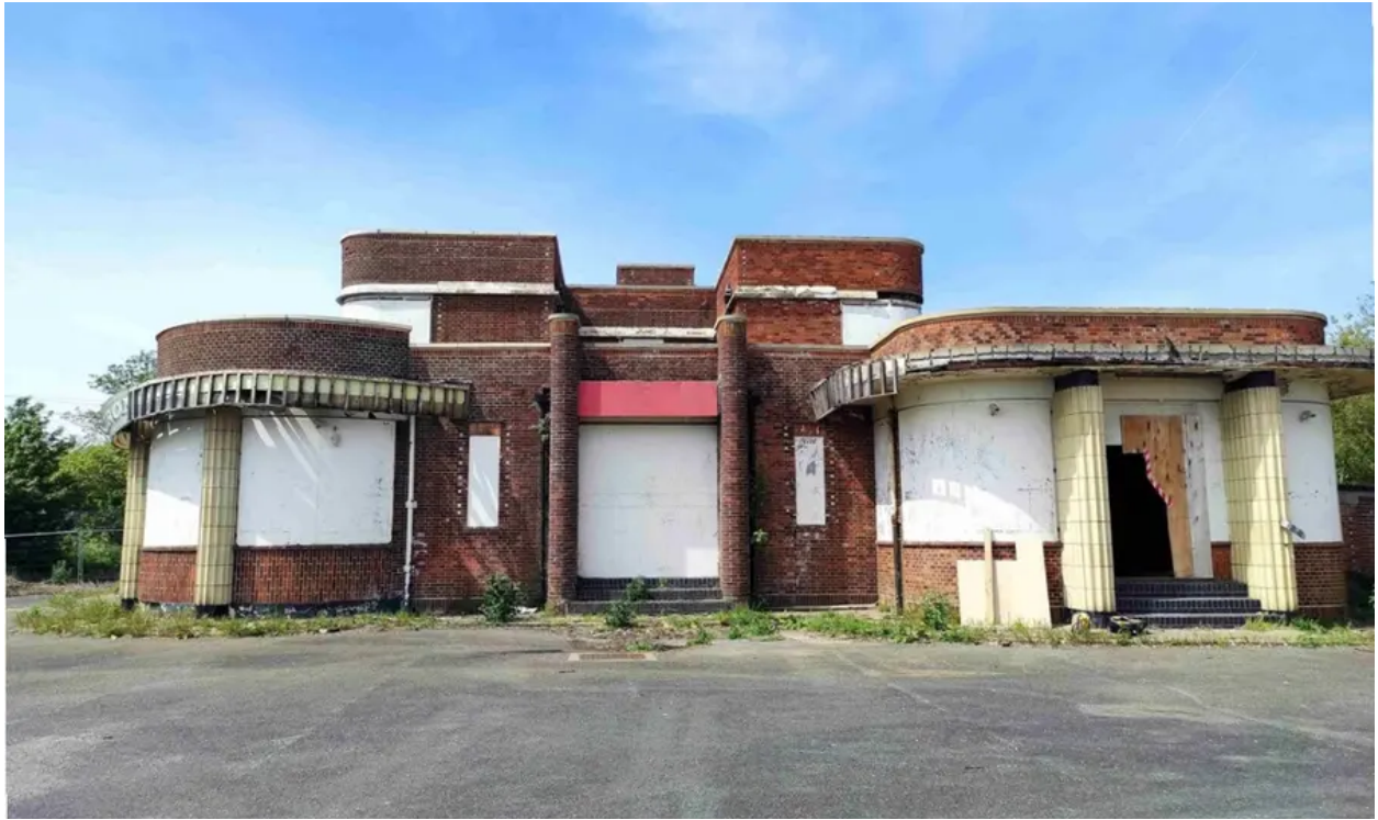
The Iron Duke, before restoration begins. Credit: Great Yarmouth Preservation Trust.
