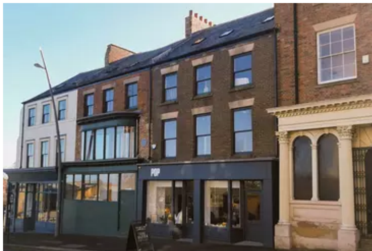
The same houses after restoration, now including a Pop Recs venue
