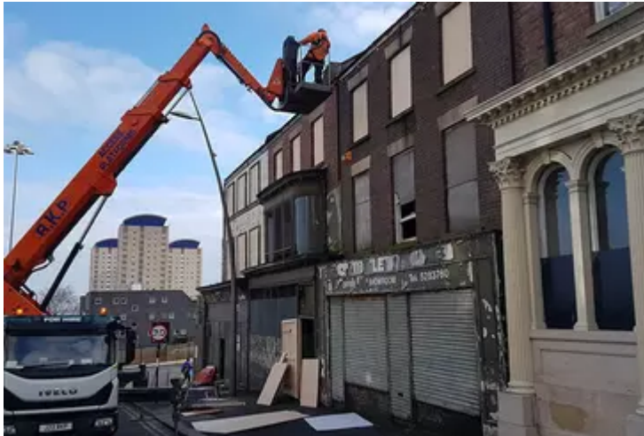
Georgian houses in Sunderland before restoration
