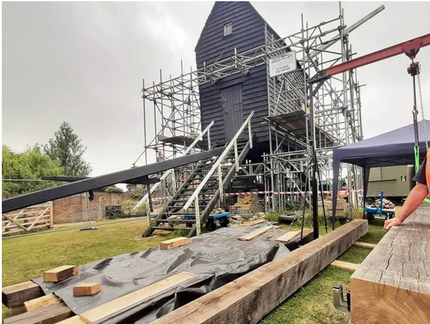
Scaffolding lifted the mill while the huge oak beams that support it were replaced.
