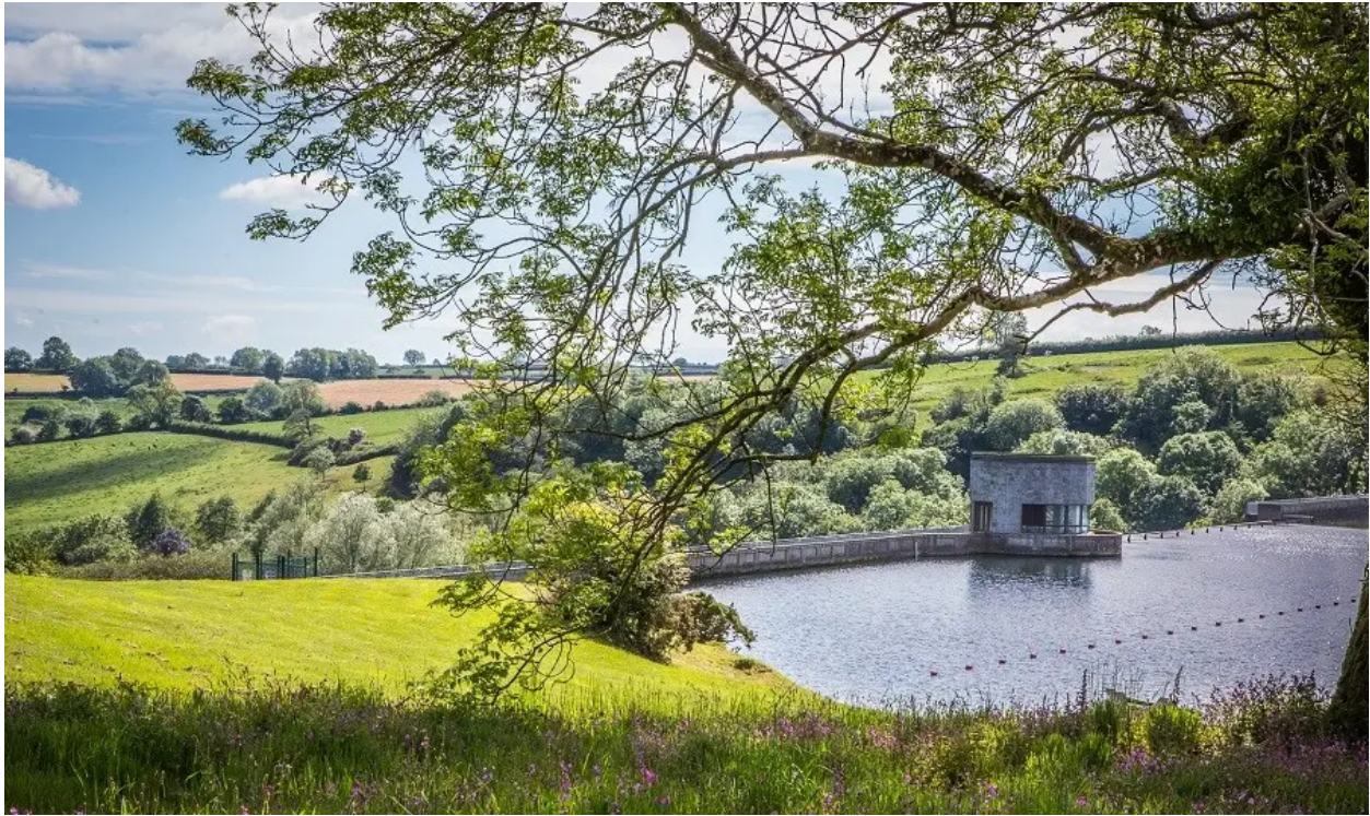
A view of Llys y Fran lake and the dam on a sunny day with a tree in the foreground
