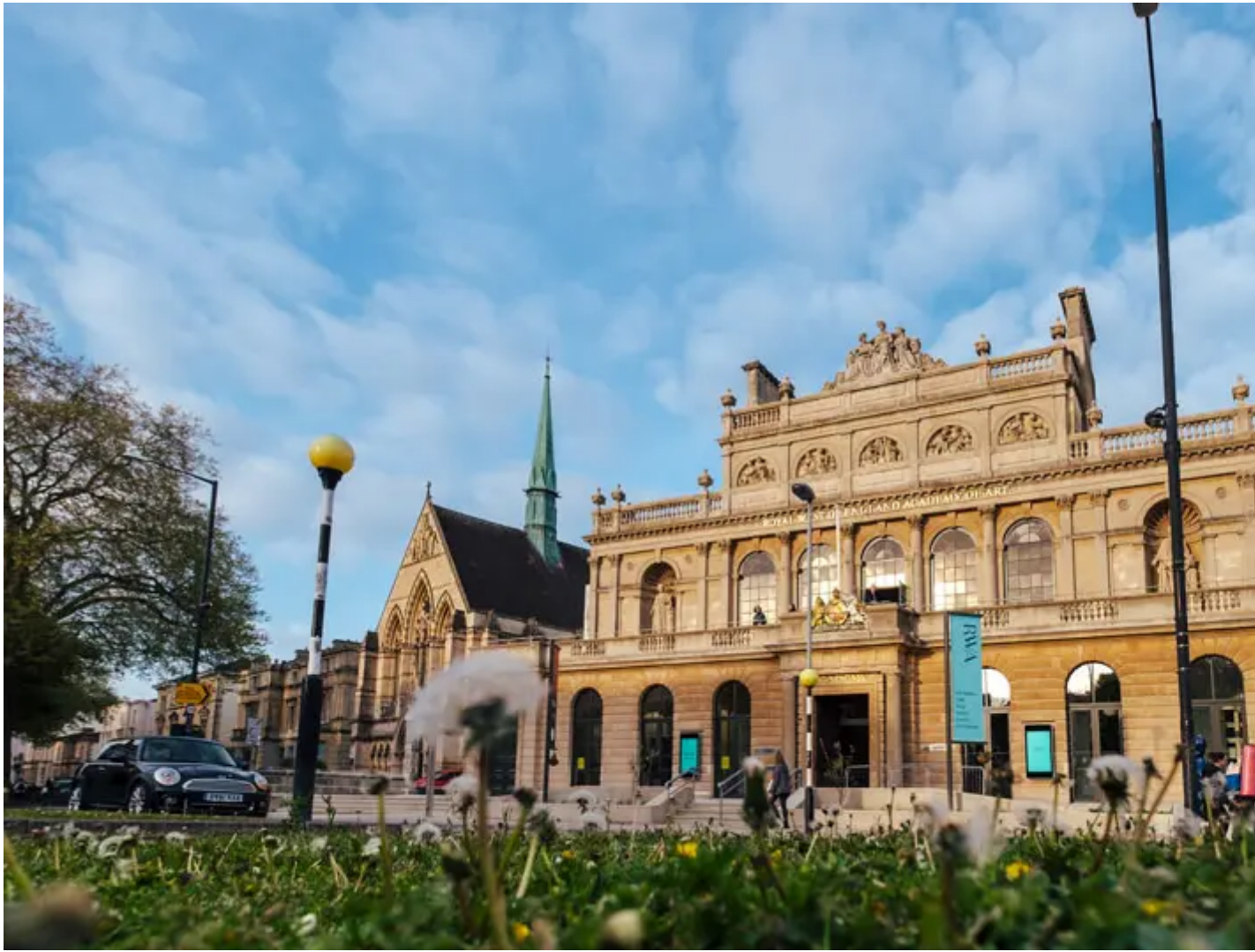
RWA exterior following capital works. Credit: Evan Dawson
