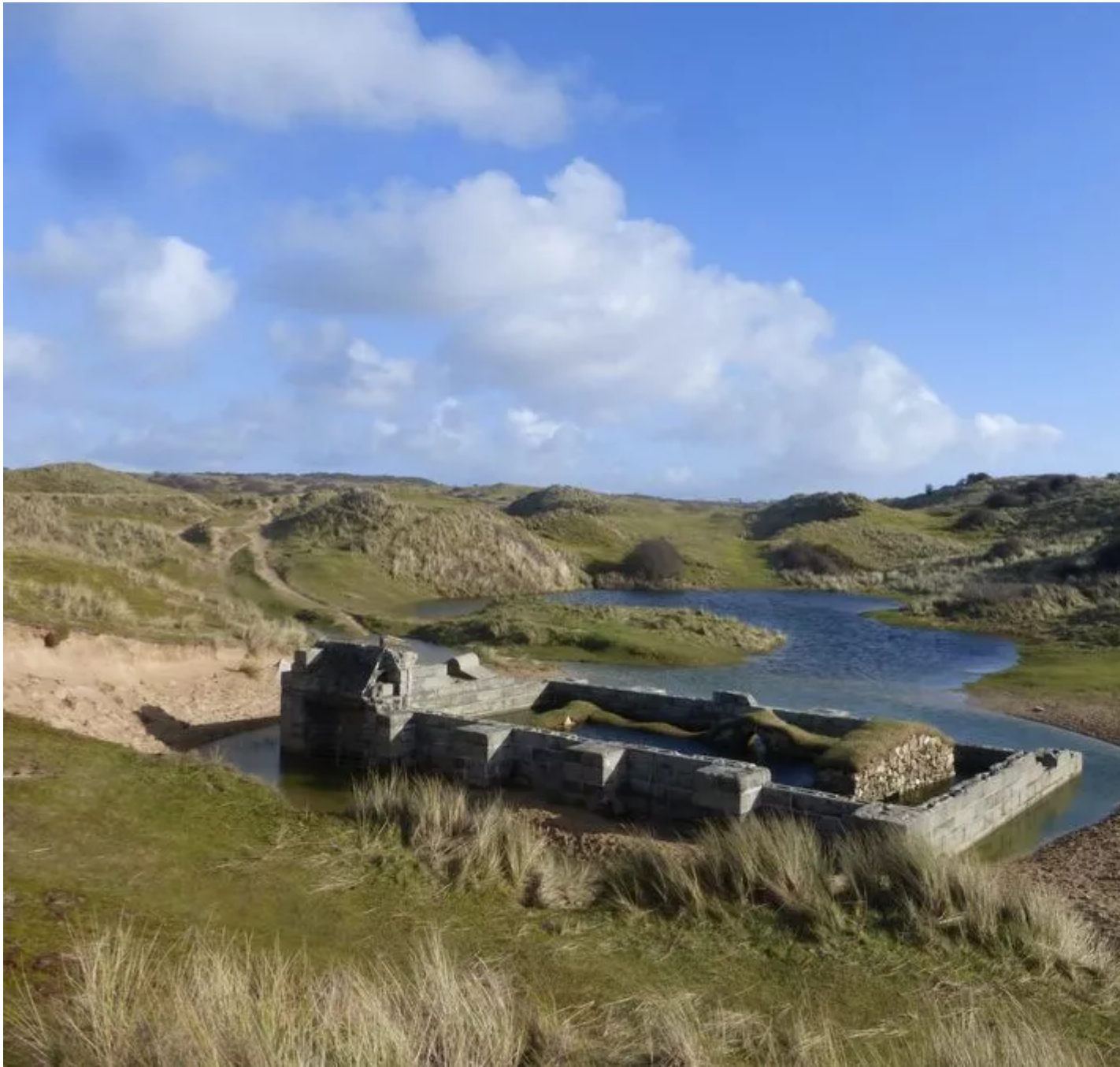
St Piran's Oratory at Penhale Sands in Perranporth flooded. Credit: Cornwall National Landscape
