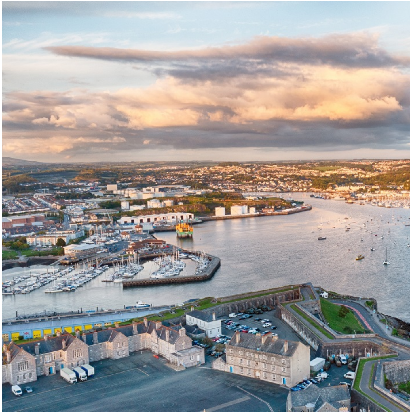
Plymouth has rich marine and coastal heritage. Credit: Chris Gorman/Big Ladder Photography.
