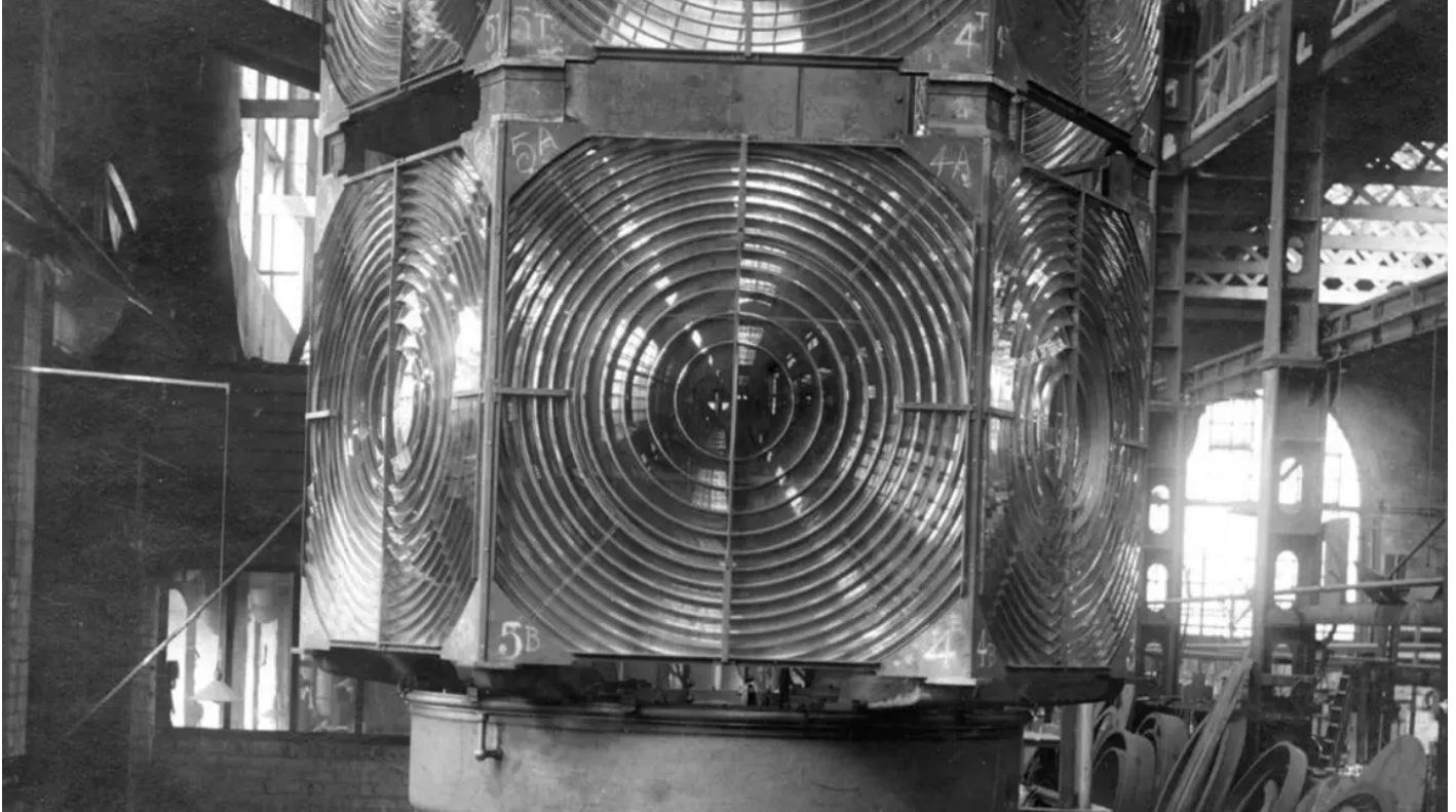
The Mew Island Lighthouse Optic is a rare hyper radial Fresnel lens. Titanic Foundation
