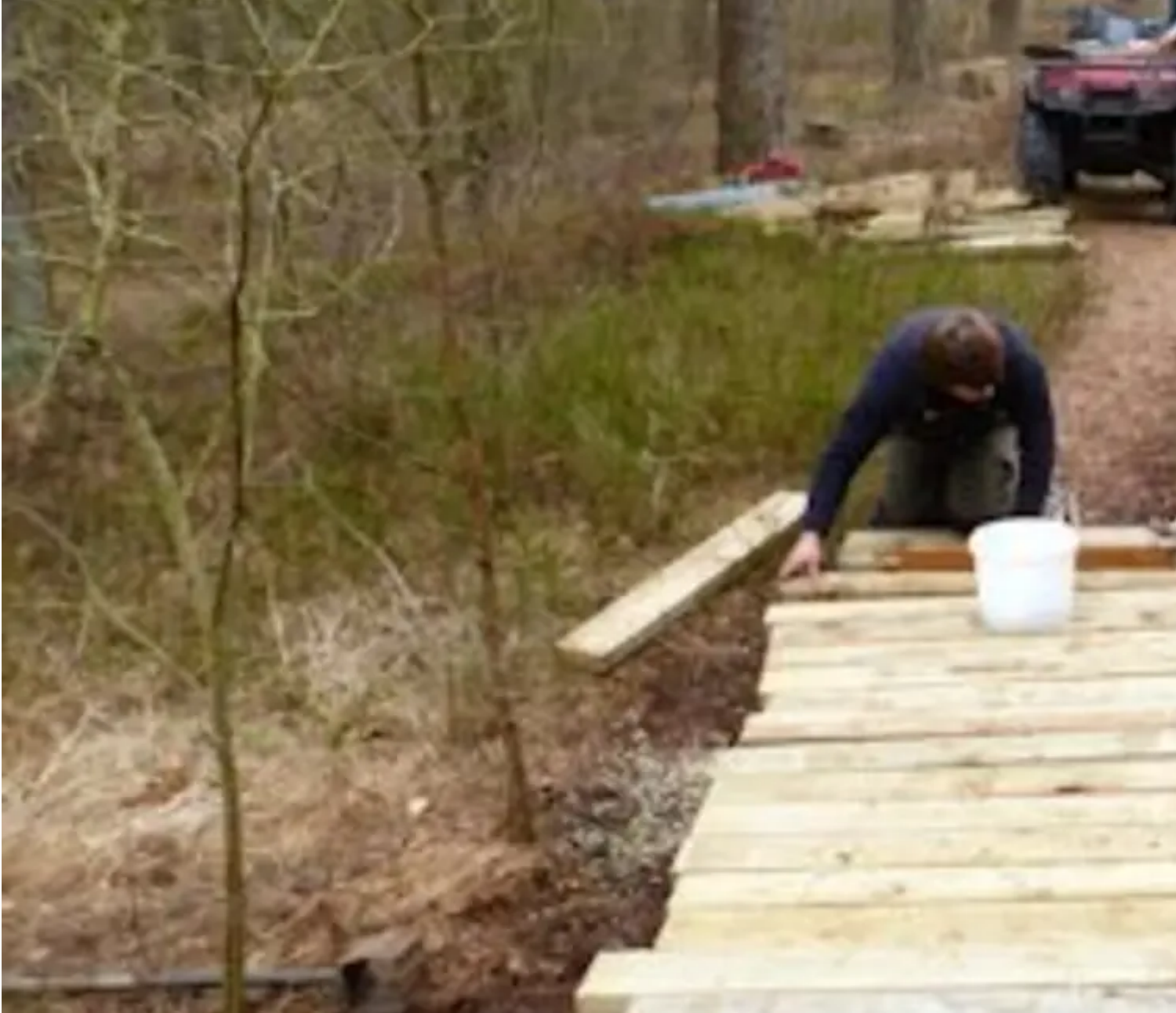
Boardwalk building at Cliburn Moss nature reserve
