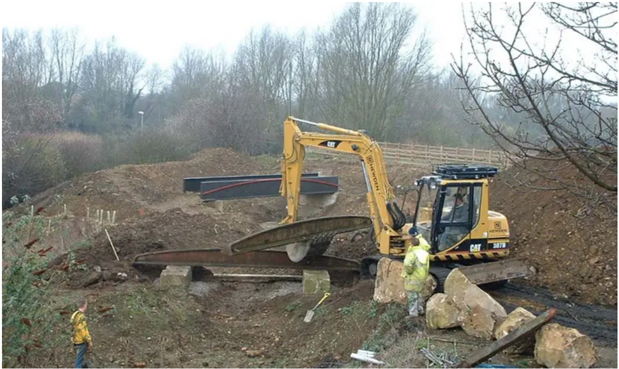
The Caterpillar Demonstration Team spent five weeks digging and landscaping the haven. Credit: Railworld Wildlife Haven.
