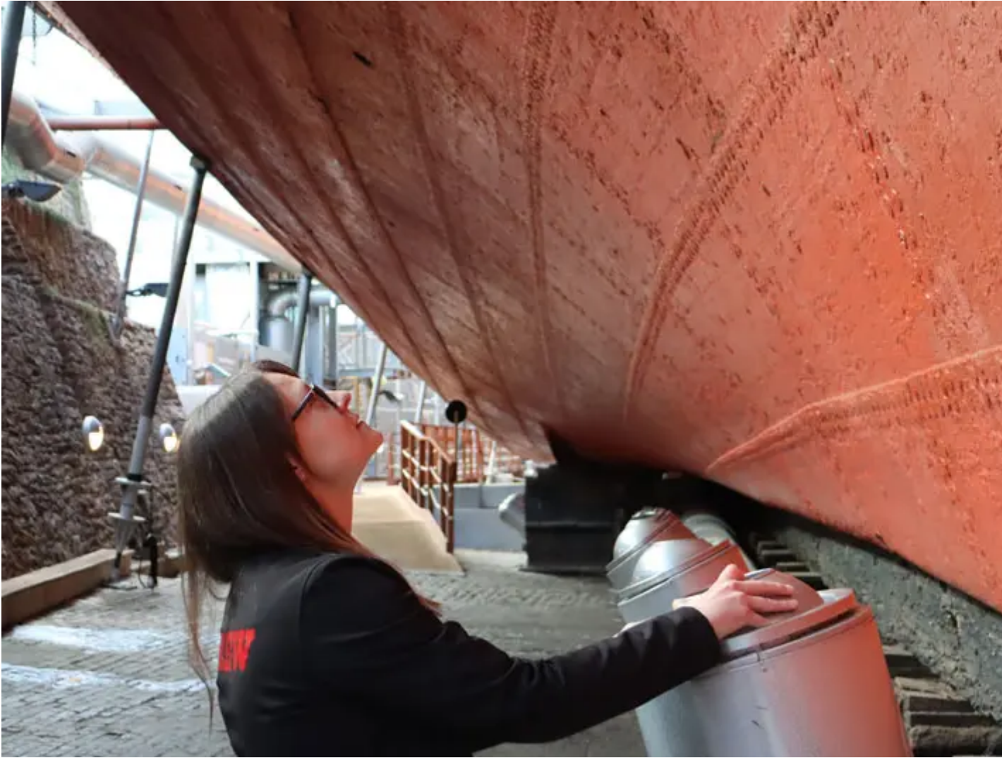
Bespoke dehumidifiers keep the fragile iron from corroding in the dry dock. Credit: SS Great Britain Trust
