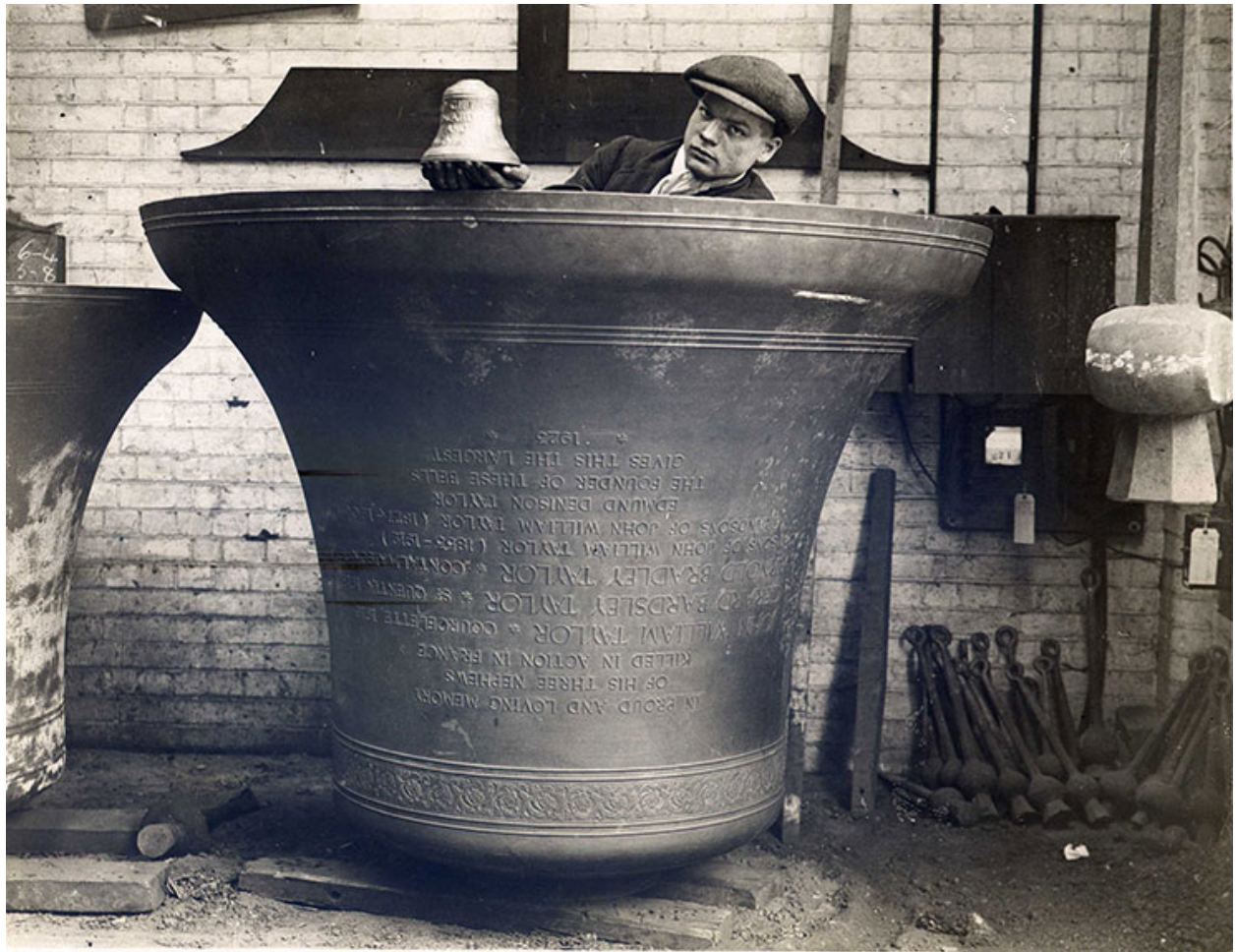
Large carillon bell created at the foundry, which has been producing bells since 1859
