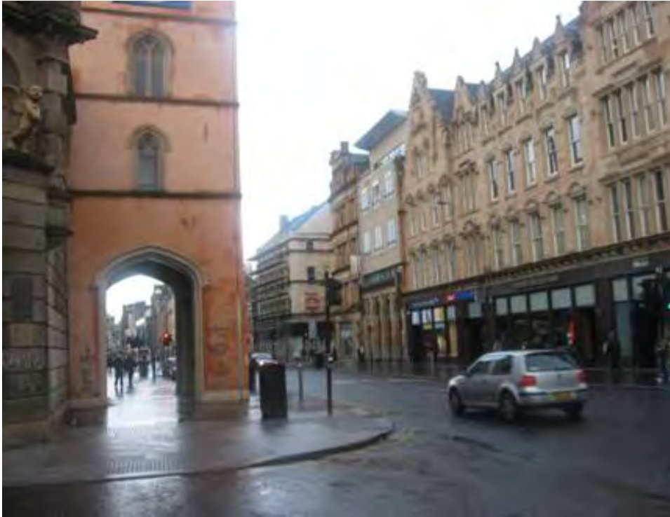
Merchant City – Trongate, showing restored buildings on both sides of the street.
