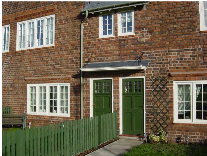
View of properties in Model Village showing quality of conservation work involving reinstatement of original detailing and joinery patterns
